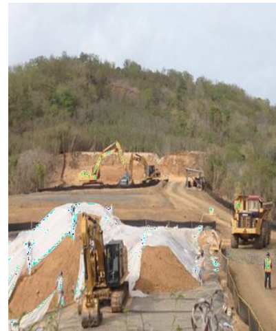
NAPR Removal Action SWMU 77
