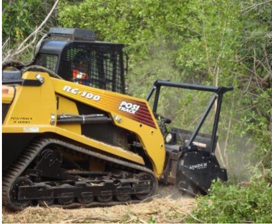
Non-Intrusive Vegetation Clearance
