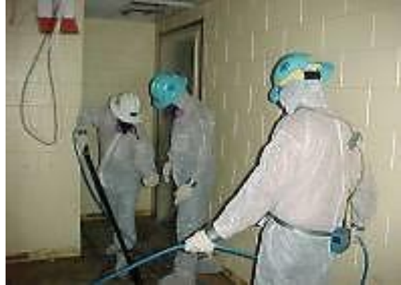
ACM removal, Dupont Agrochemical Plant.
