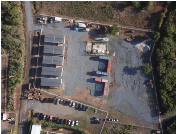
Camp Garcia Facility Construction
