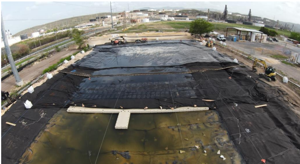
Liner Wet Installation
