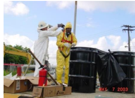
UST Clean-up Roosevelt Roads Naval Station
