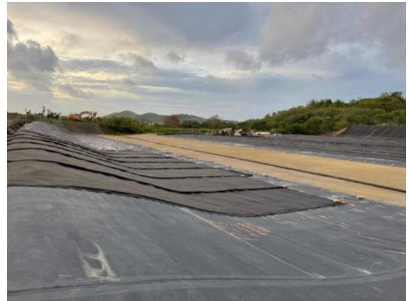
EC Waste Liner Installation
