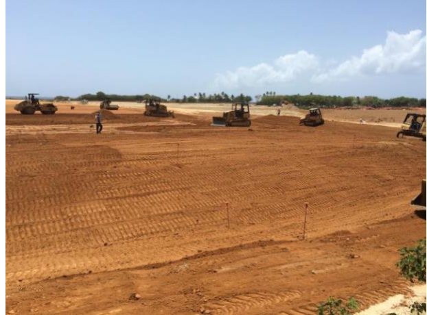
Clay Cap Installation On Landfill Closure
