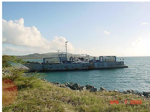
Mobilization into NASD, Mosquito Pier, Vieques, UST Closure OP1, fuel facilities and UST's.
