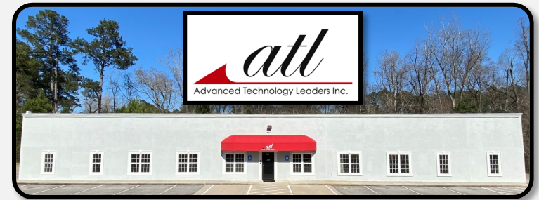
Modernized Classroom Facilities located in Martinez, GA
